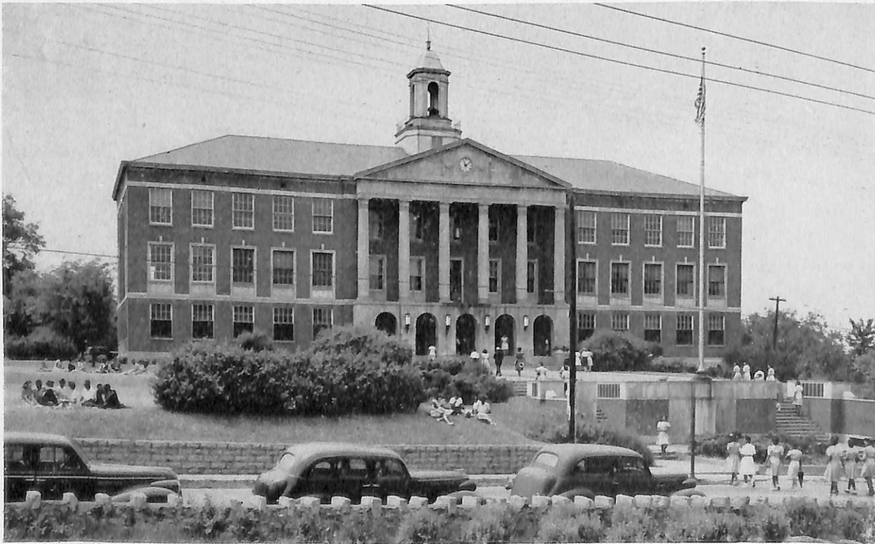
Administration Building, Tennessee State College
