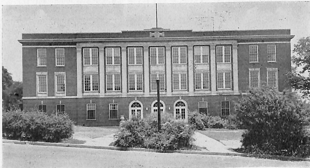
Harned Hall, Science Building, Tennessee State College
