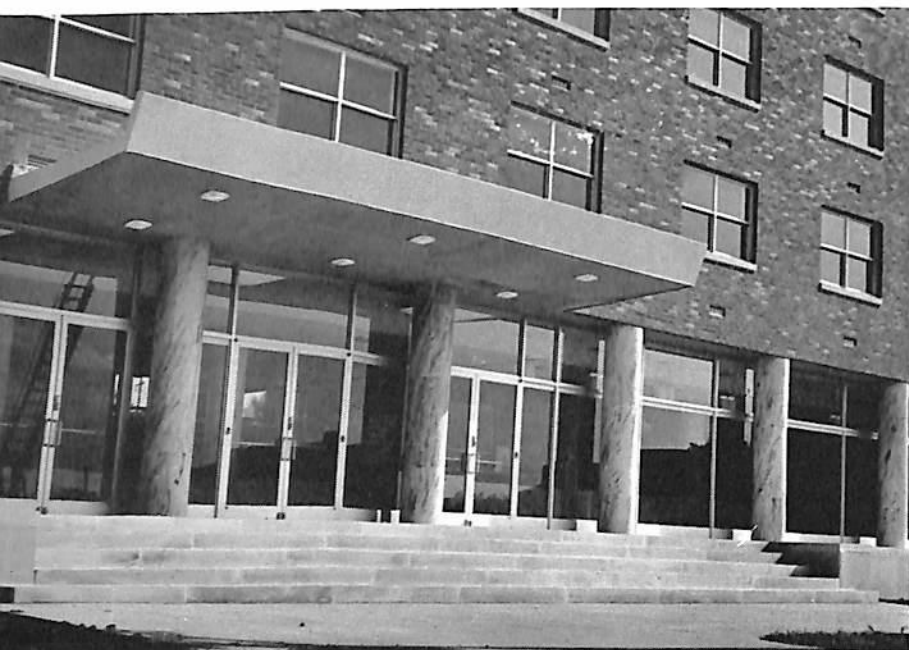
The Building—Lena B. Watson Hall
