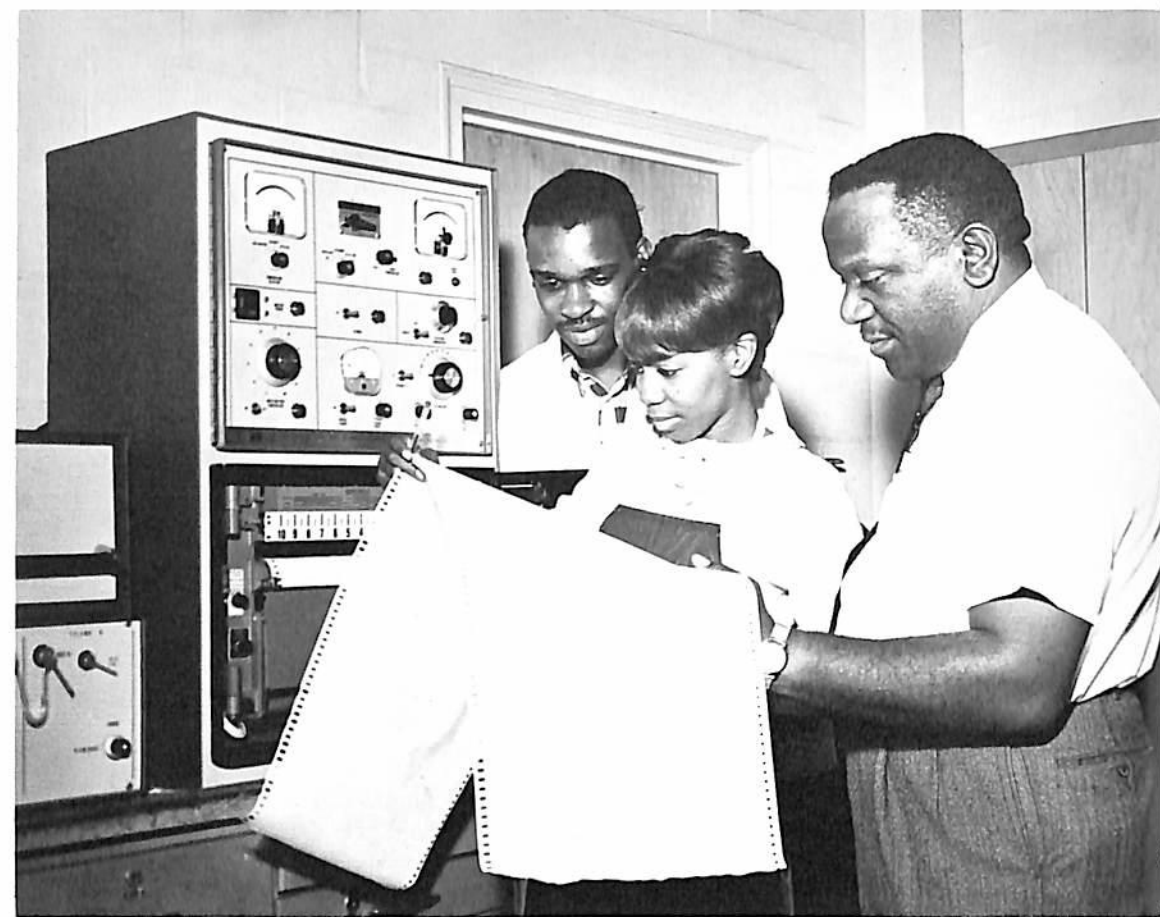
Chemistry professor, Dr. Lonnie Haynes, assists analytical chemistry students Jacqueline Hill and James Phillips in the study of a gas chromatograph which they are using to determine the number of components in an organic mixture.
