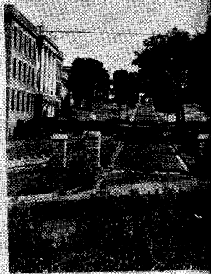
WEST ENTRANCE SWIMMING POOL
