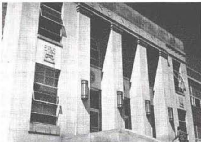
Home of the campus engineers
