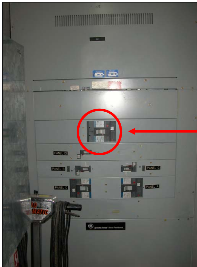
Pictured above: Main breaker panel in Room 121
