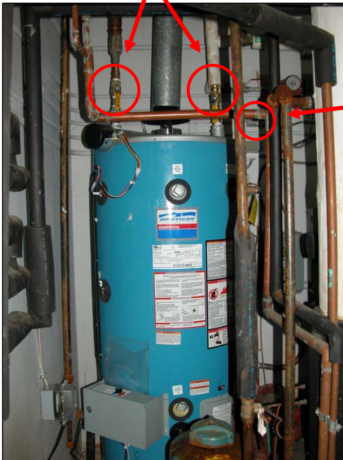
Water supply (in and out) valves
