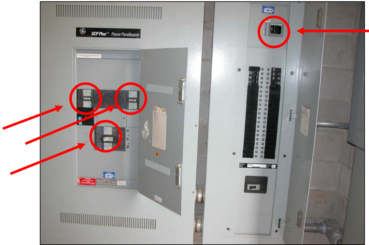
Pictured above: breaker panels located in greenhouse boiler building.
