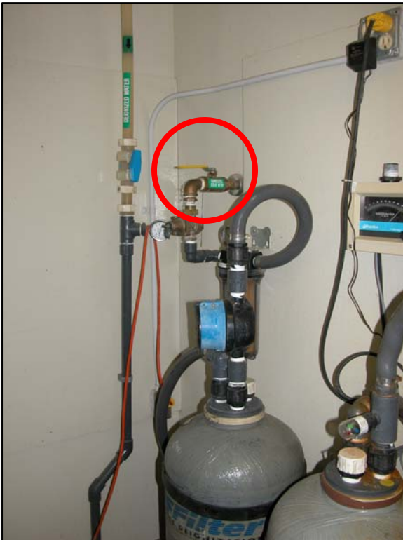
Valve to turn off water supply to deionized water loop.
