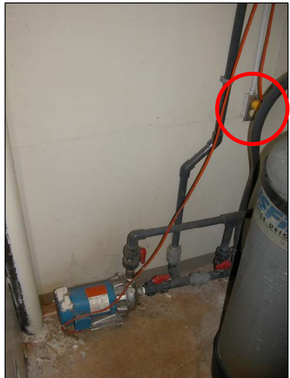
Plug to turn off circulation pump in deionized water loop.
