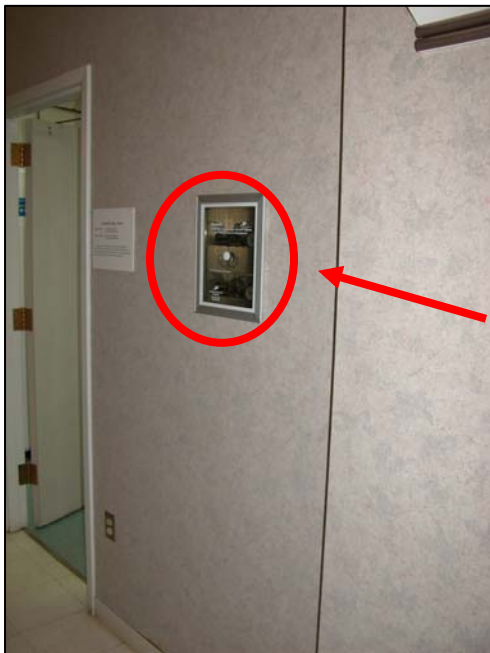
Between Rooms 111 and 115
